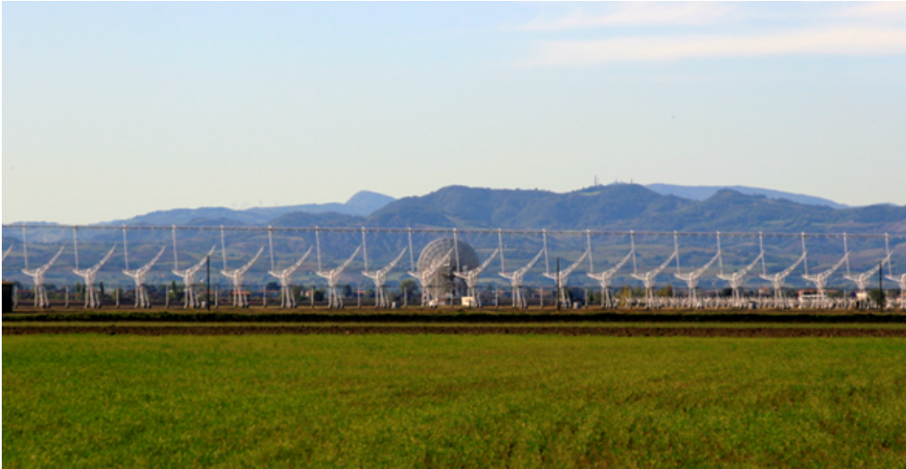
Fig. 2. A partial view of the East/West branch of the Northern Cross radio telescope, pictured from the North.
