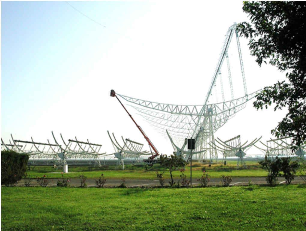
Fig. 1. A portion of the East/West branch of the Northern Cross radio telescope. Two technicians aboard a platform are checking the mirror, made up of about 1200 km of closely spaced metal wires, stretched from one end to the other.
